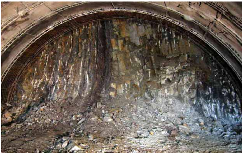
Fig. 2. Tunnel face with typical distribution of strata
