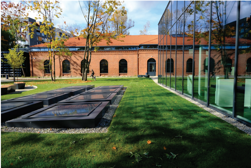
Il. 5. Building after adaptation – skylights integrated into the garden area (author of photography: Zofia Kazimierak-Piotrowska)
