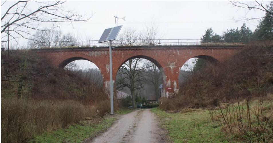
Rys. 3. General view of the viaduct B
