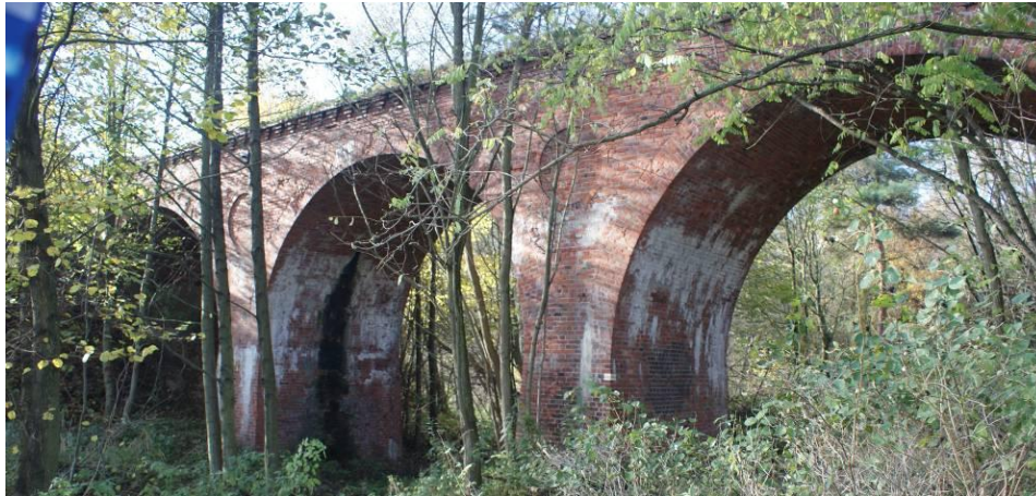
Fig. 2. General view of the bridge structure A
