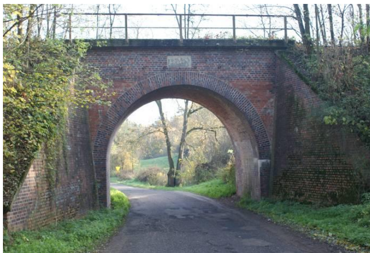
Fig. 5. General view of the bridge D
