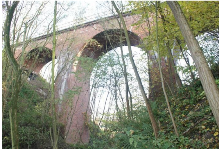
Fig. 4. General view of the bridge C
