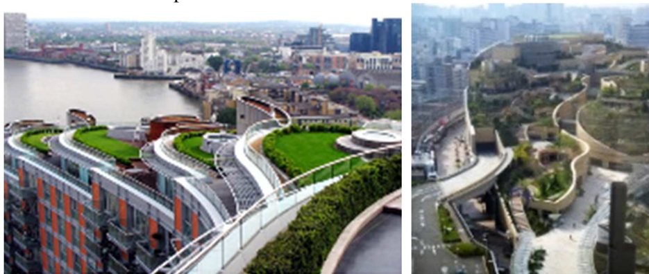
Rys. 3. Zielony dach: a) New Providence Wharf, Londyn, GB [ http://www.zinco-green-roof.com ], b) Namba Park, Osaka, Japonia [ inhabitat.com ]
