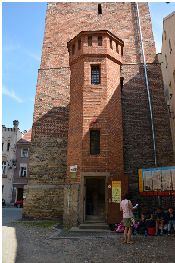
Fig. 2. View of a part of the tower and outbuilding
