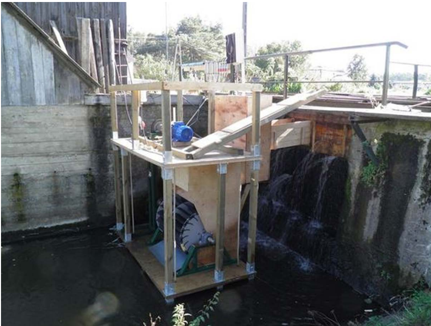
Fig. 5. Complete test stand, with a turbine enclosed in plywood housing, installed at the dam [Włodzimierz Sawicki, 2010]
