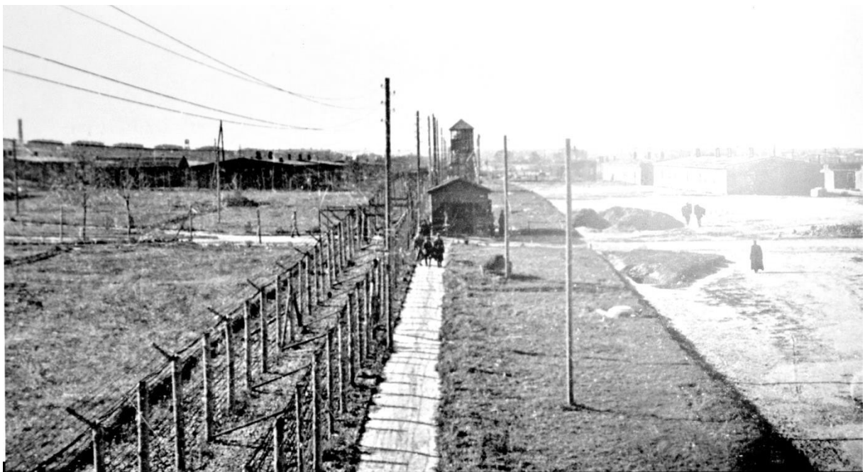
Figure 3. The camp at Majdanek after liberation in autumn 1944. - view of the western fence of the prisoner section with the original overhead power line visible (reproduction of the plaque from the exhibition at the State Museum at Majdanek).
