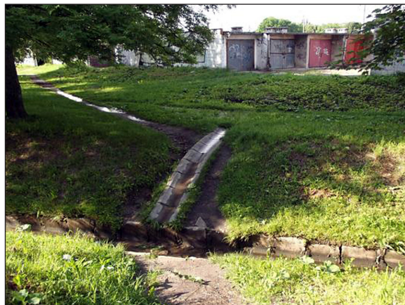
Figure 2. Wastewater discharge from garages area into the studied receiver (III sampling point)
