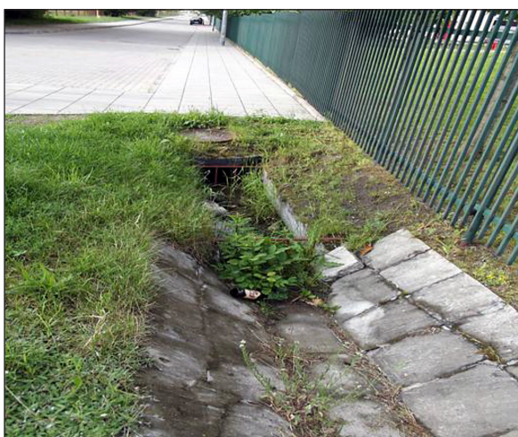
Figure 3. Wastewater discharge into the sewer drain (IV sampling point)
