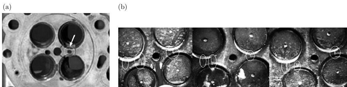
Fig. 11. The cracked diesel engine cylinder head: (a) Takahashi et al. (2010), (b) Li et al. (2013)
