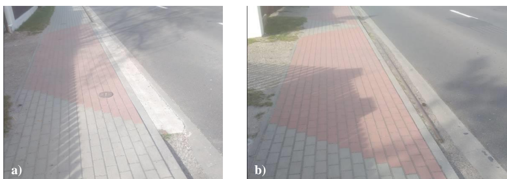
Fig. 5. "Facilitation of passage" through triangular gutter: a) concreting, b) steel pipes
