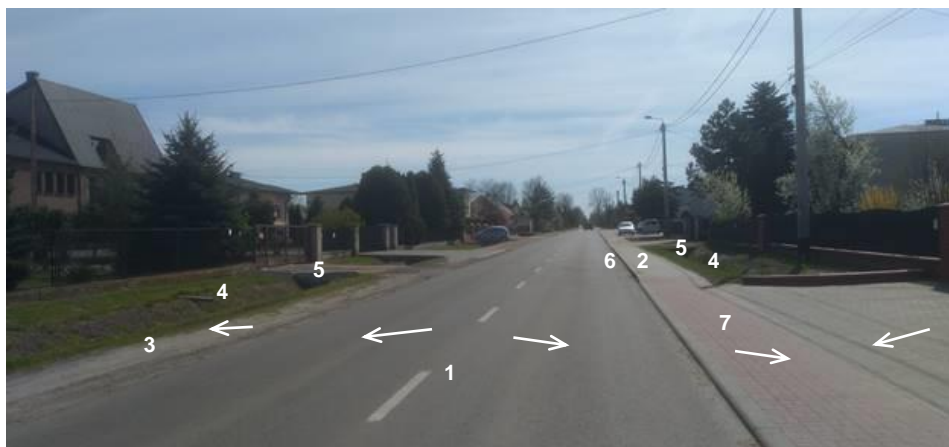
Fig. 1. Elements of drainage in built-up area, arrows indicate the direction of water runoff: 1 – road surface with a „roof-like slope”, 2 – sidewalk, 3 – unpaved roadside, 4 – ditch, 5 – culvert, 6 – near-curb gutter, 7 – exit with lowered curb
