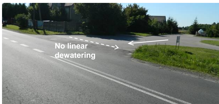
Fig. 8. Possibility of covering the road surface with water from the paved area – the problem would be partially solved by using a box-gutter at the exit
