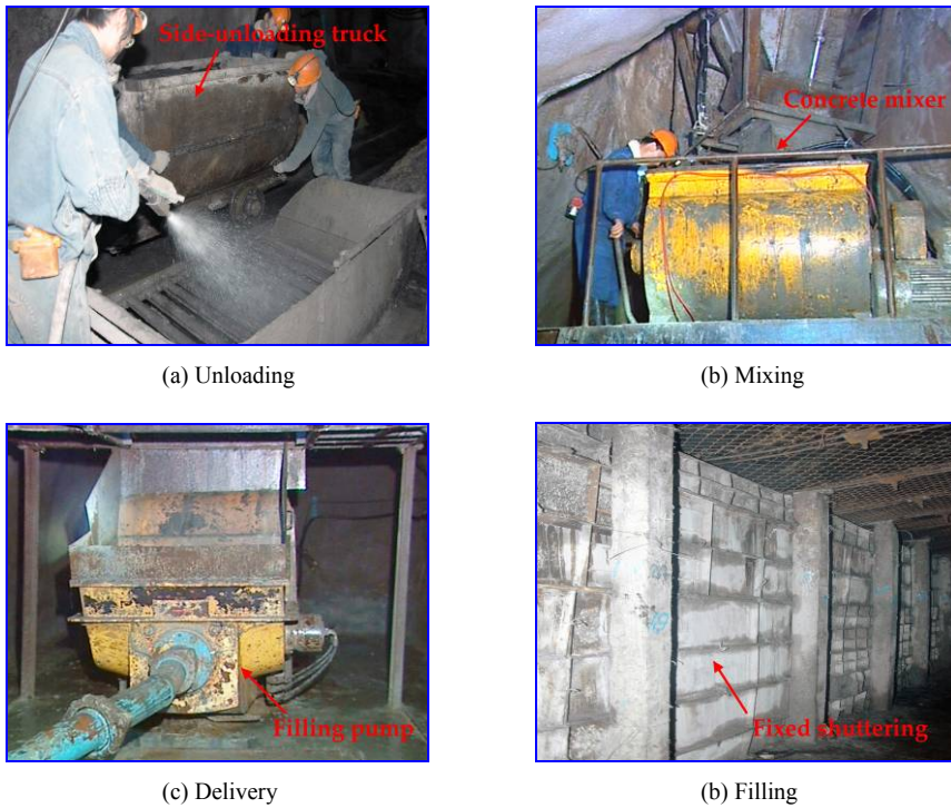
Fig. 8. Site construction process
