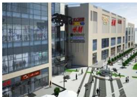
Fig. 17. ... and after the modernisation
