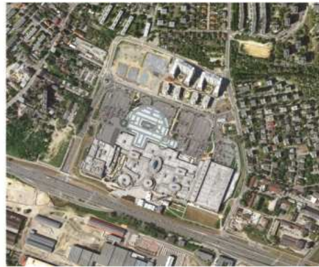
Fig. 11. SCC in Katowice.
