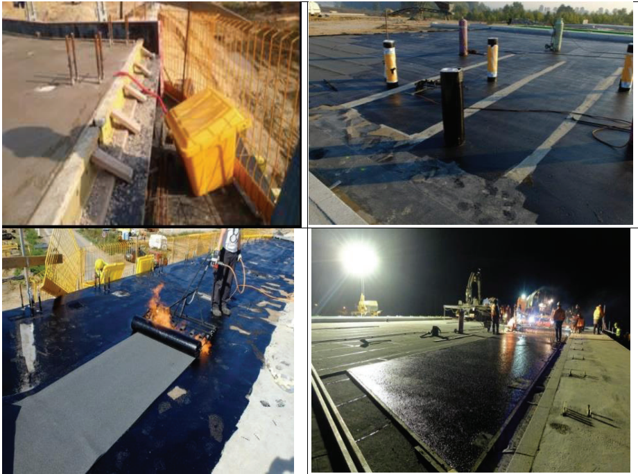
Fig.4 The pavement construction. Sensors fixed inside the deck and put into the box, which contained the data acquisition devices. Visible location of the sensors on the surface; they'rey stripes on a primer black background.
