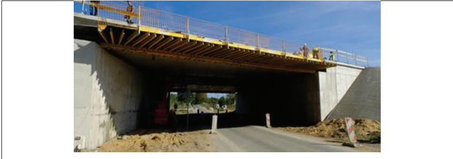
Fig.2 The view of the bridge deck at the A2 carriageway under construction.
