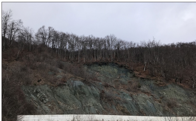
Figure 5. Landslide along the road segment (no. 1 at Fig. 1)
