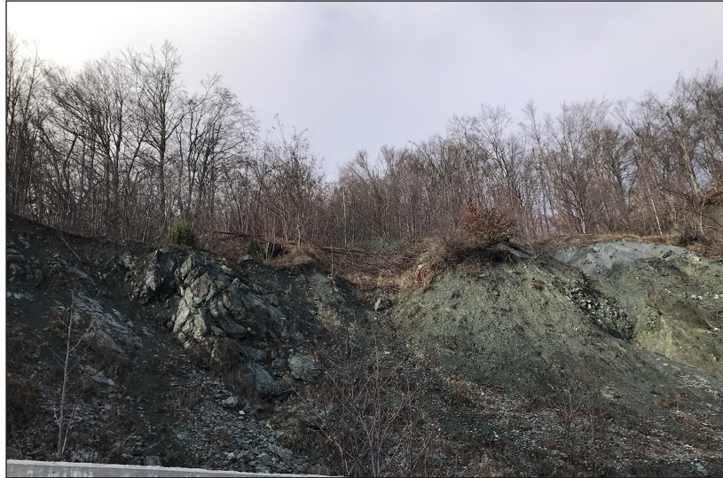
Figure 6. Landslide along road segment (no. 2 at Fig. 1)
