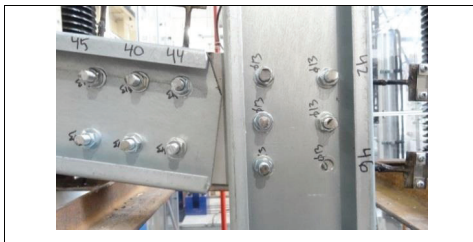
Fig. 10. Failure mode of specimen M12C15025I10
