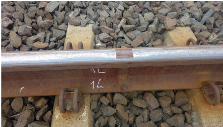
Fig. 1. View of the contactless joining of rails made by thermite welding
