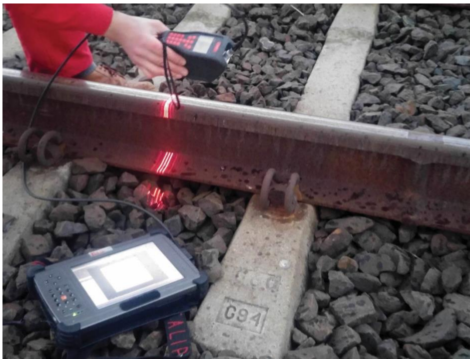
Fig. 4. View of the measurement with the Calipri laser device of the rail head profile 60 cm in front of the non-contact joint of thermite-welded rails, the laser module in one of the seven measurement positions – the top
