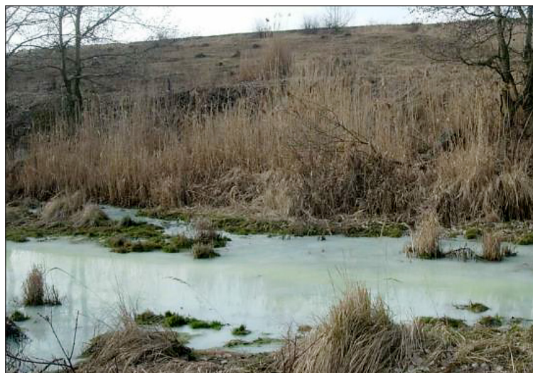
Fig. 2. Leaks of hydrogen sulfide waters from the drainages of the eastern part of tailings storage facility No. 1
