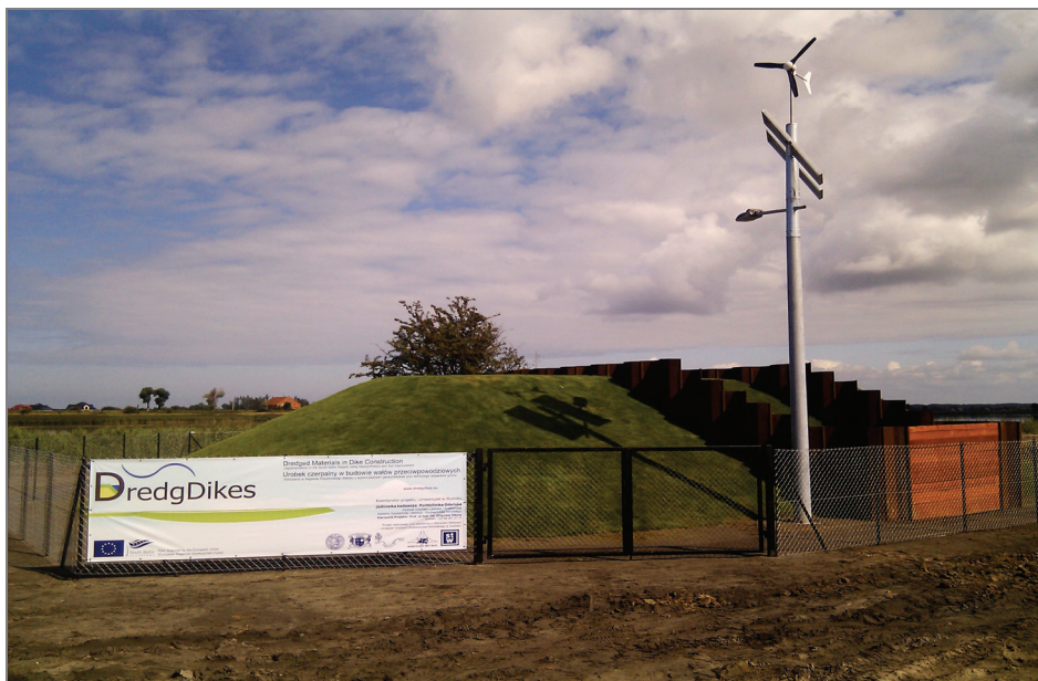
Fig. 1. View of the test dike
