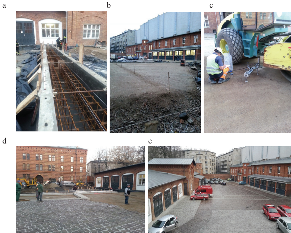
FIGURE 1. State Fire Department in Kraków manoeuvring area's remodelling: a – trenching and constructing the structure of linear drainage; b – constructing the primary base from aggregate; c – primary base testing; d – laying the surface cobblestone layer from porphyry; e – the end result
