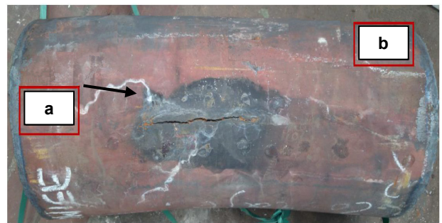
Fig. 2. (a, b) The areas from which samples were taken for mechanical properties testing: a) damaged area, b) not damaged area
