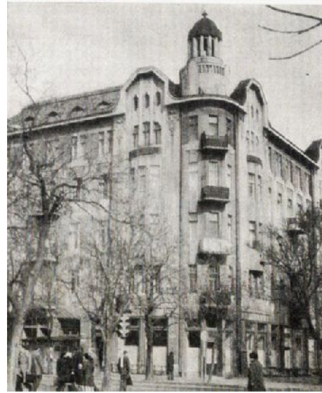
Fig. 2. Chernigov and Shestopal's Revenue House, corner cupola. Photo from book Odessa. Architectural-historical note . V. Timofeenko, 1984.
