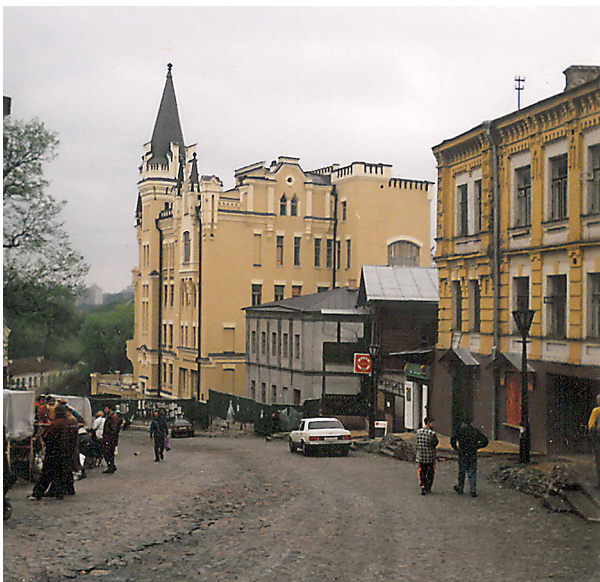
Fig. 4. Residential house at 15 Andriyivsky Uzviz Str. Photo by Julia Ivashko, 2017
