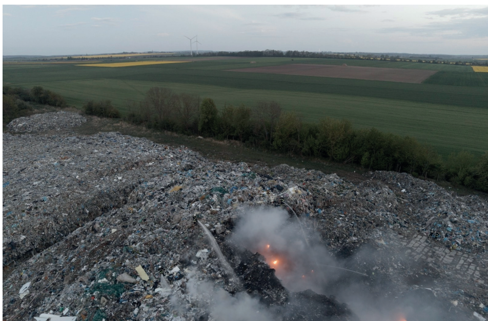
Figure 1. Landfill fire – image from RGB camera of Yuneec H520
