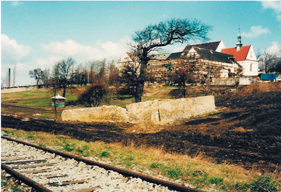
Photo 9. View on the Reformati Monastery during its renovation after a disastrous water flux in the transverse heading Mina
