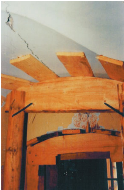
Photo 3. Fragment of supported roof of the monastery
