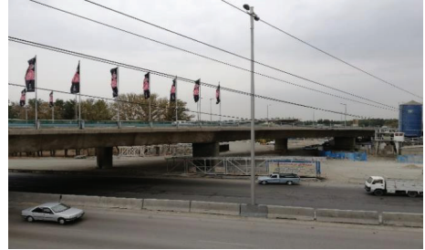
Figure 2. General view of the Hesarak Bridge.
