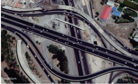
Figure 1. Aerial photo of the Hesarak Bridge [15].
