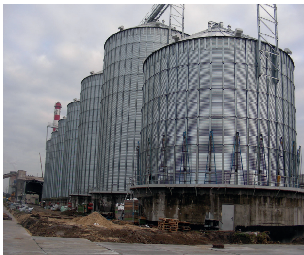
Fig. 9. General view of the silos from the west
