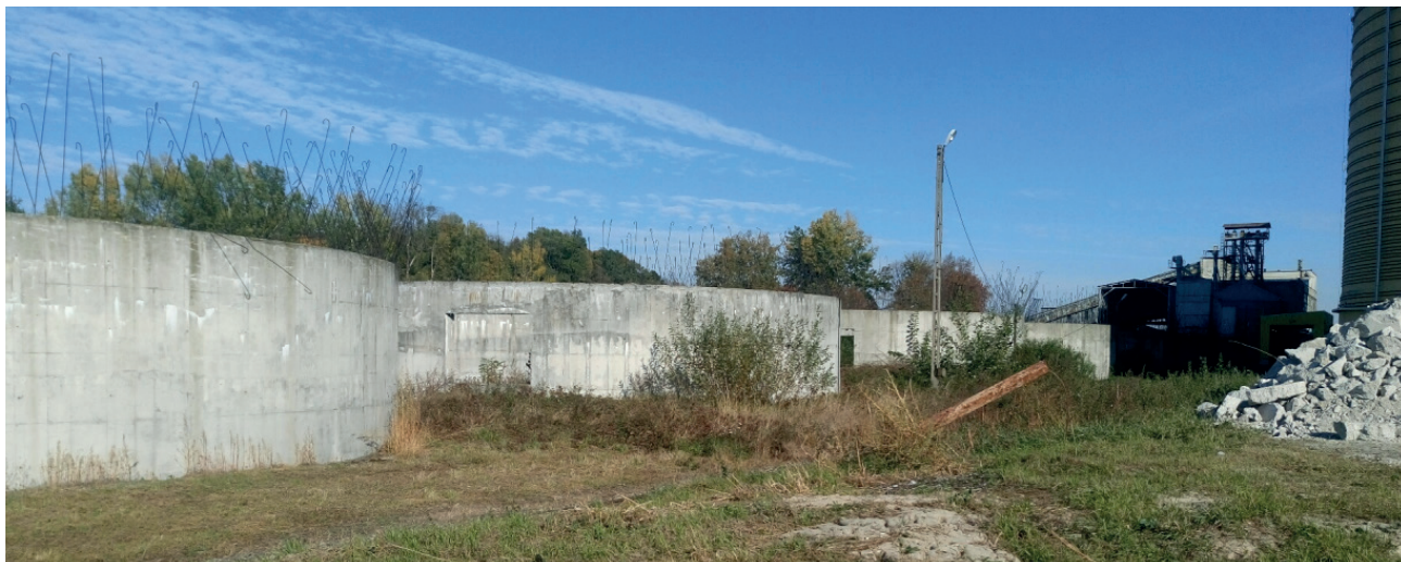
Fig. 1. General view of the foundations for the silos from the south
