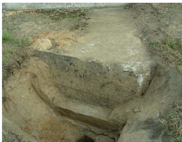
Fig. 2. The exposed foundation plate No. 7
