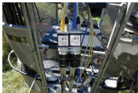
Fig. 2. Basler acA1300 monochrome cameras mounted in a mobile elevated work platform (MEWP)
