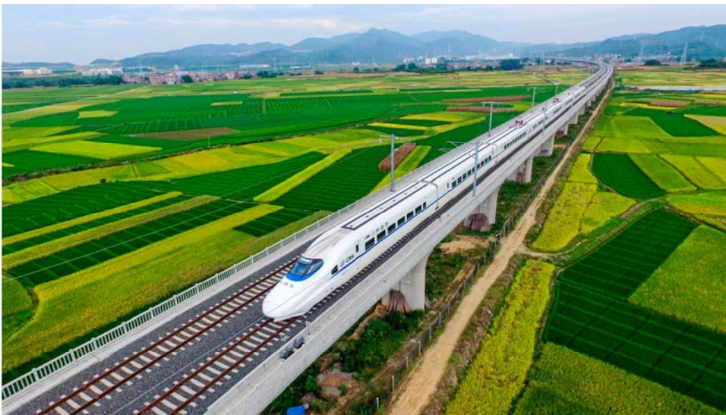
Fig. 9. High speed rail on bridge. More effective, less impacting the environment and less expensive than railways on the ground. Source: Picture by Wei Wanzhong in Dagens Nyheter, 10th September 2016.
