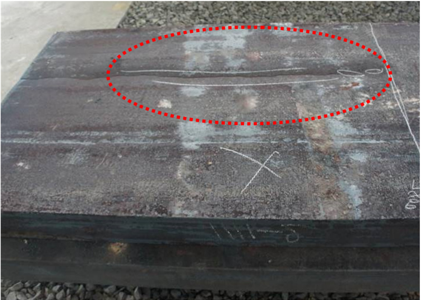
Fig. 9. A longitudinal surface crack on inside radius
