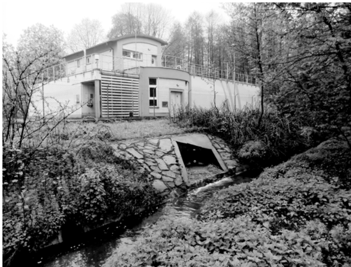
Fig. 4. Sewage treatment plant with an outcome into a small water resource
