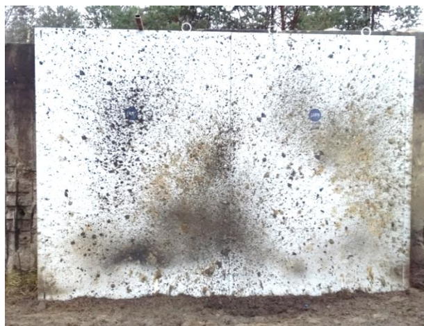
Fot.11. Fasada po próbie - II etap Photo 11. Facade after the trial of the II stage
