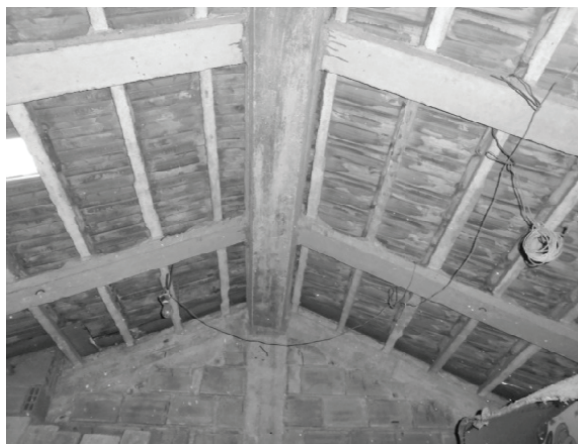
Fig. 17. Covering Structurally Supported by Prefabricated Beams
