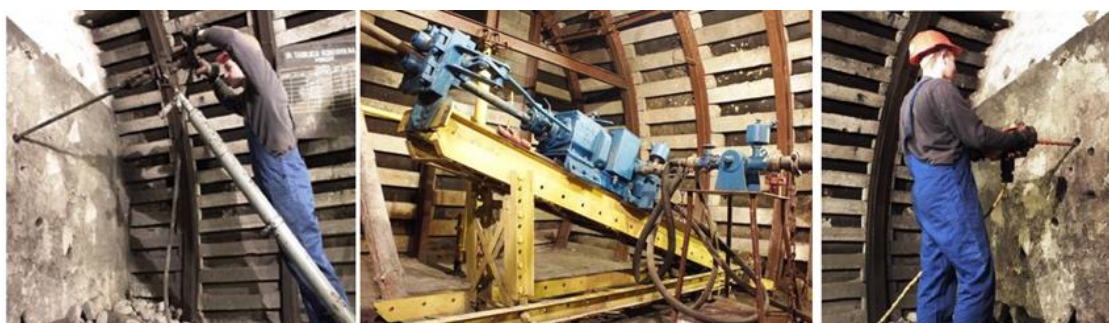
Fig. 4 Drilling of blast holes
