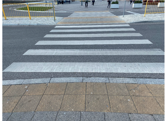
Fig. 12. Tactile pavement in a hazard zone (along the carriageway edge). A correct, ridge-less connection between different pavement textures. Kielce. Photo: M. Wijas
