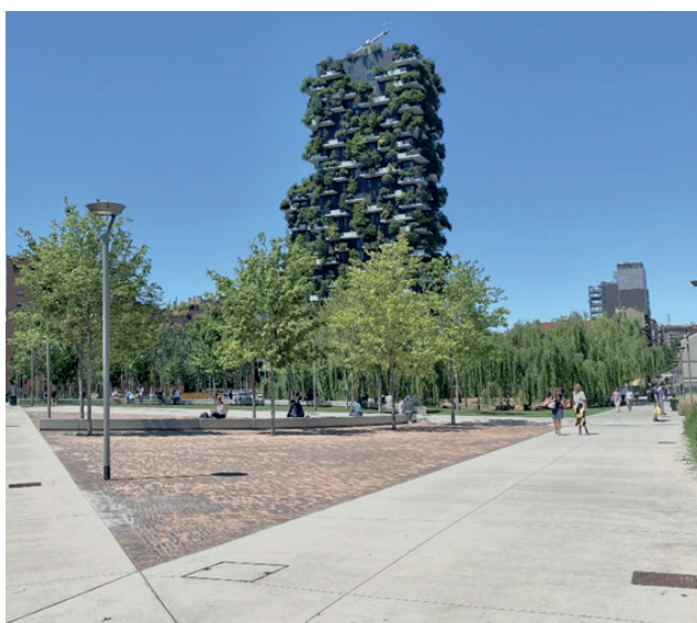
Fig. 20. A ridge-less connection of different pavements that constitute the Porta Nuova square in Milan, Italy. Photo: M. Wijas
