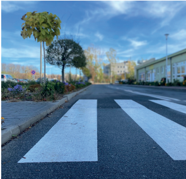
Fig. 15. An incorrect transition between a carriageway and a sidewalk at the location of a pedestrian crossing. Opole. Photo: M. Wijas.
