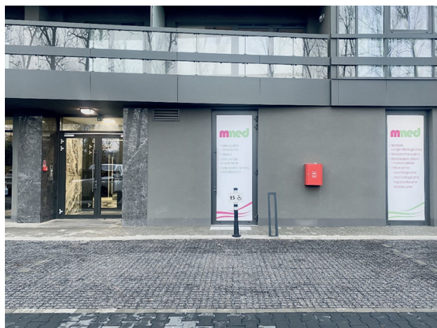
Fig. 13. Unsuitable pavement and incorrect marking of a parking space for disabled persons. Kielce.
