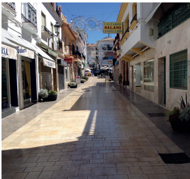
Fig. 1. An example of a correctly implemented path on both sides of a pedestrian zone. Spain. Photo: W. Tracz
