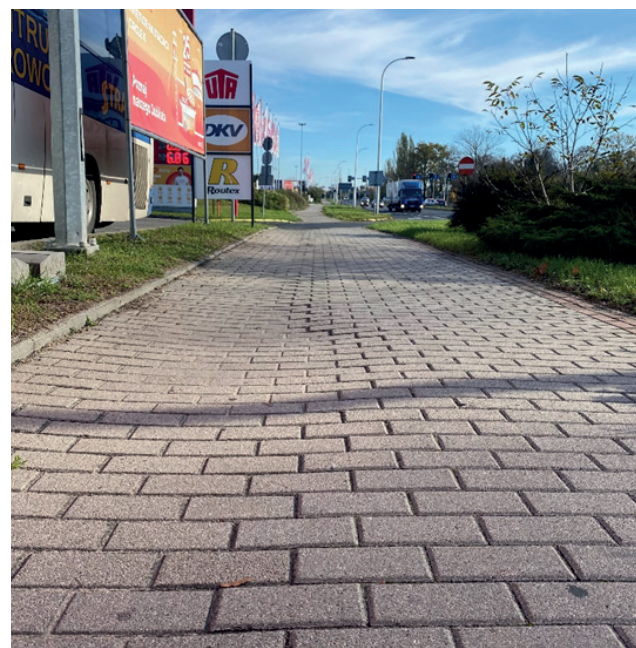
Fig. 18. A barrier in the form of deformed sidewalk pavement. Opole. Photo: S. Mochocka
