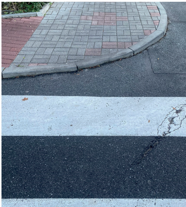
Fig. 16. An incorrect transition between a carriageway and a sidewalk at the location of a pedestrian crossing. Opole. Photo: M. Wijas
