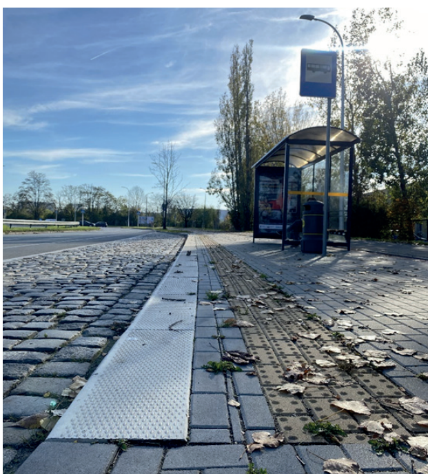
Fig. 8. The correct use of tactile pavement at a bus stop. Opole. Photo: S. Mochocka
