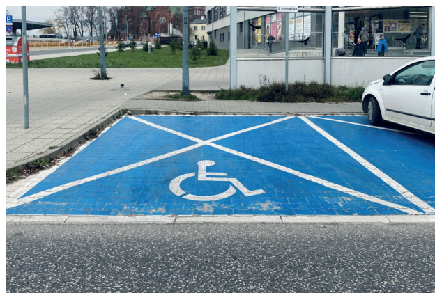
Fig. 14. An example of the correct marking of a parking space for disabled persons. Ridge-less connection with the carriageway and sidewalk via a 2 cm ridge. Appropriate pavement colour and type. Kielce.
