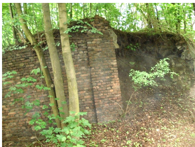
Fig. 1 A wall constituting a remnant of the Hugo zinc smelter buildings
