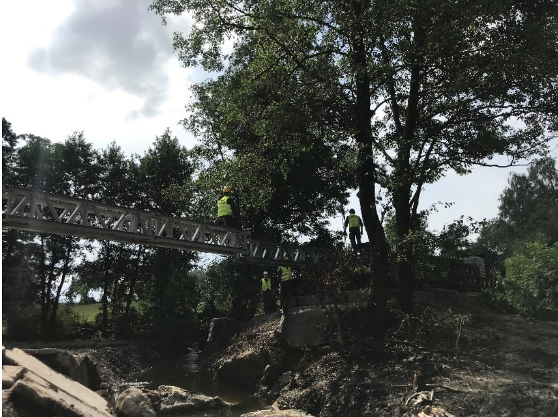
Figure 5. Connecting sections of the structure in the described technology.
