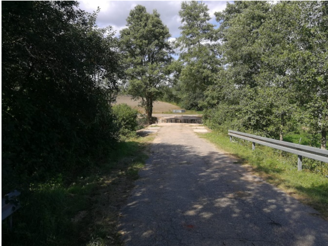
Figure 4. Field conditions at the crossing point.
