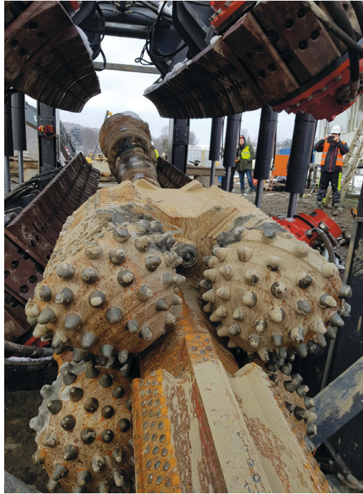
Fig. 4. Roll reamer inside the pusher pipe [collection of J. Janicki]
