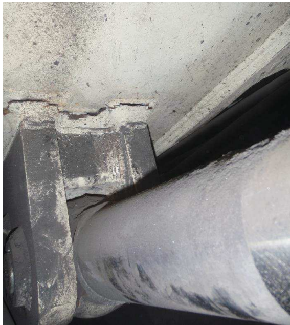
Fig. 1. Damages to the welds connecting the lifting eye system of the tilt cylinder with a gob shield sheathing sheet [12]
