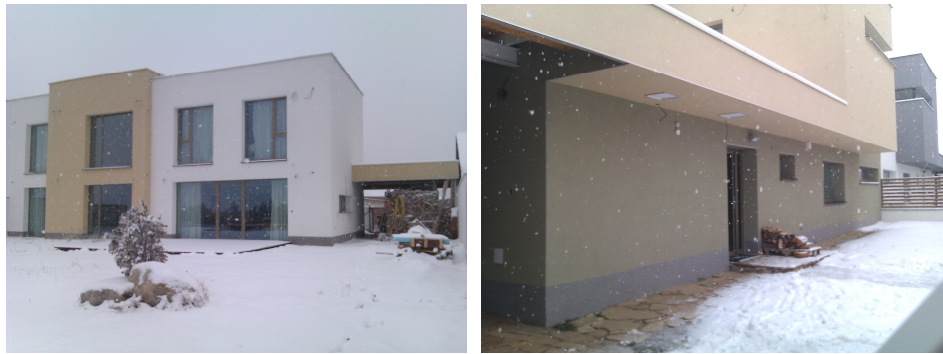
Fig. 4. Views of the building - family house
