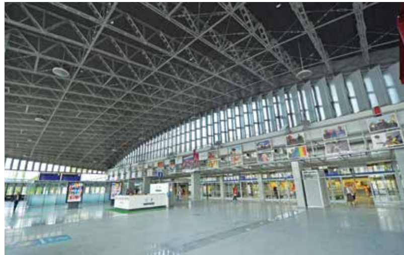
Photo 2. Cash hall Warsaw East Station. Photo PKP S.A.
