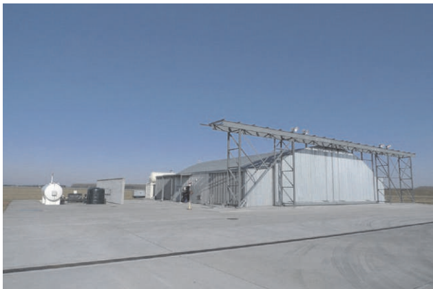
Fig. 8. Hush house in the 31st Tactical Air Base in Krzesiny
